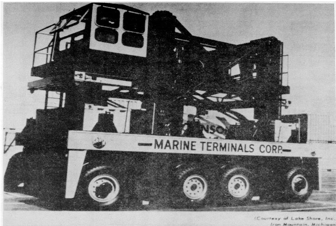
Figure B-2. Shoremaster.
